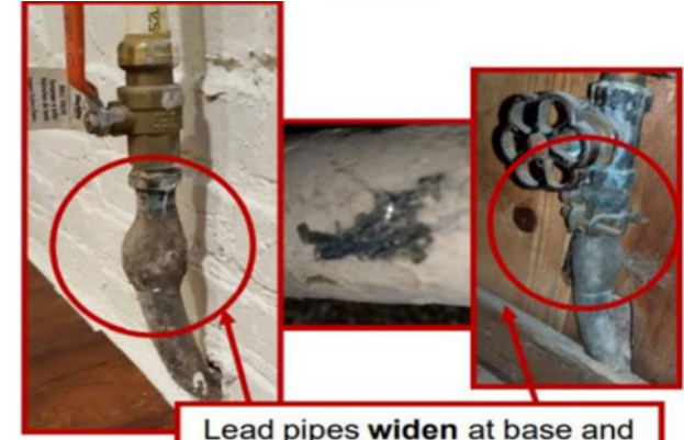
Lead pipes widen at base and often form a "bulb."
